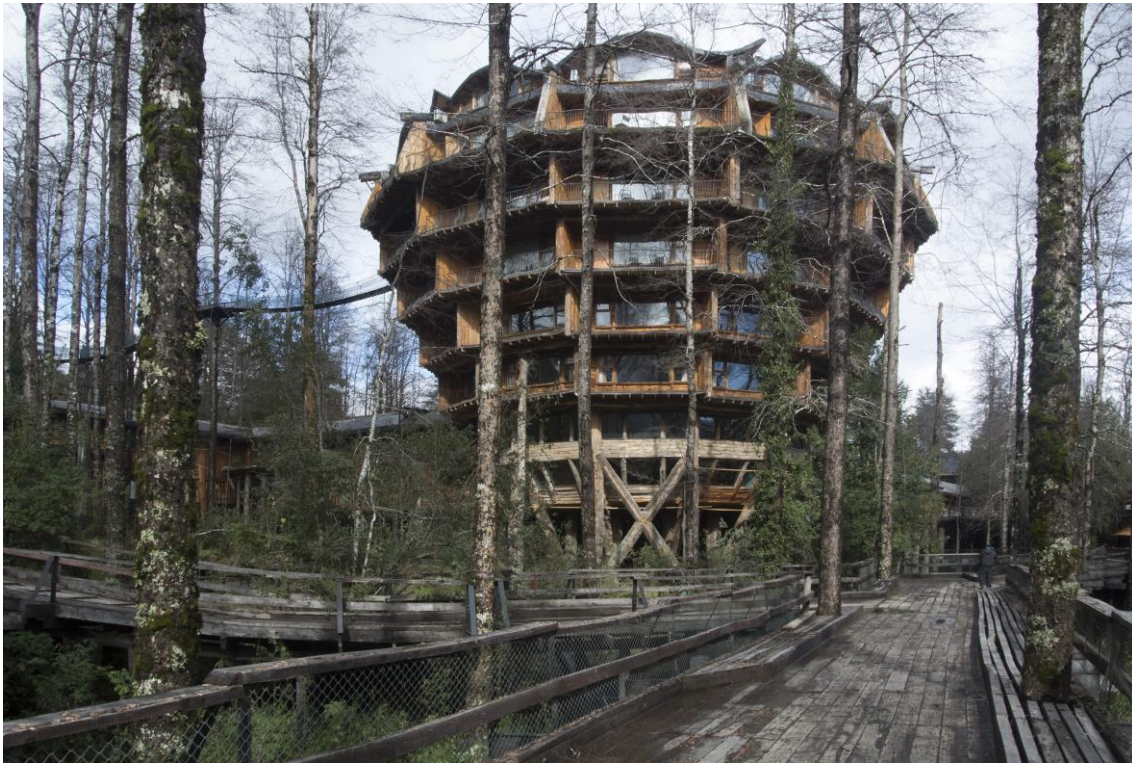
Figure 6 - View of Baobab Hotel from the bridges
